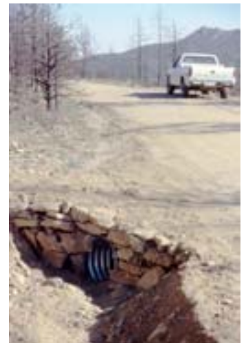
To be effective, culverts must be installed properly and at proper locations.
