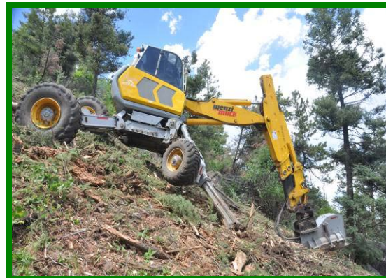
All-terrain excavator with forestry attachment
